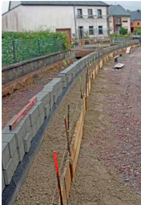
Fig. 11: Concrete placement during the construction of a gutter system
