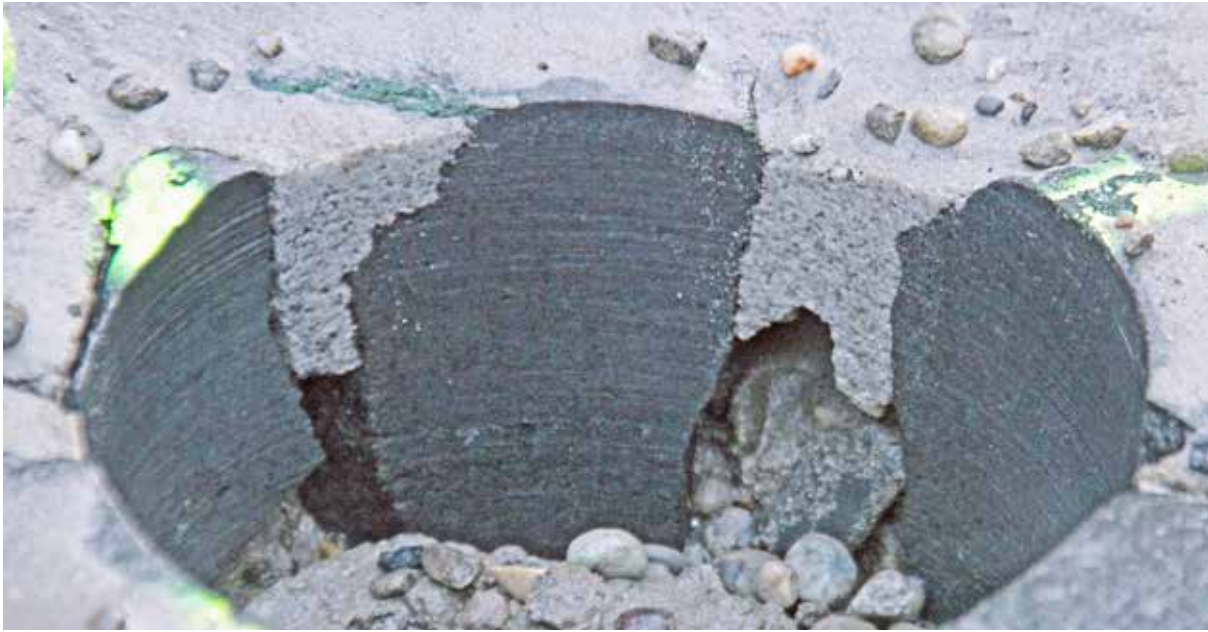
Fig. 2: Absent bond between the quarry stones and the jointing mortar
