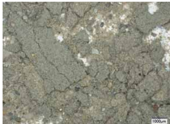
4 Damage pattern 1: contamination on the block surfaces (on the left, contaminated block surface/on the right, gained con- taminant)
