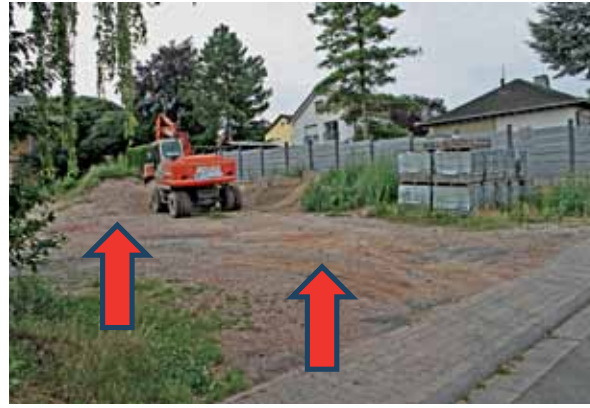
3 Damage pattern 1: ambient sources of contamination
